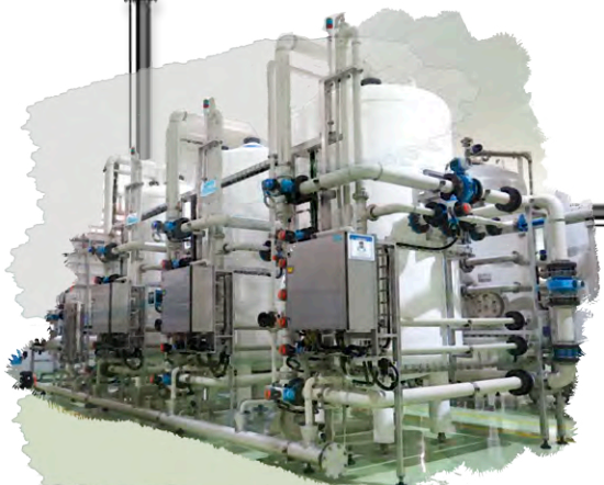
5 Water Treatment System
