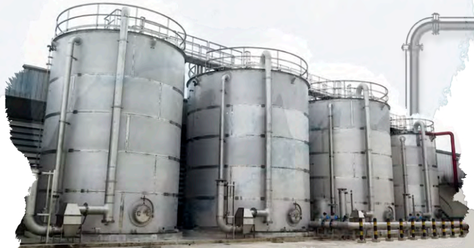
3 Water Storage Tank
