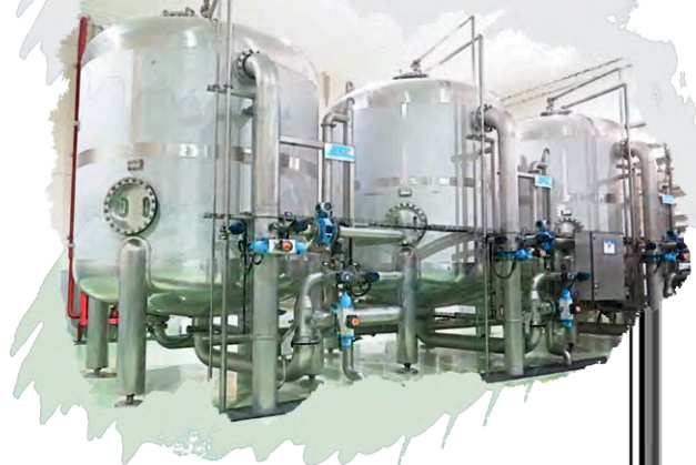
2 Pre-Water Treatment System
